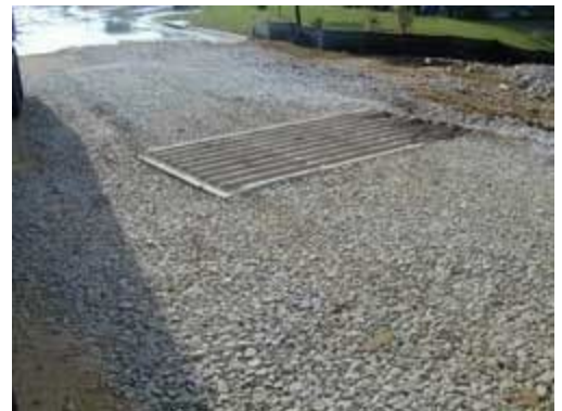
Stone Construction Entrance with Washrack
